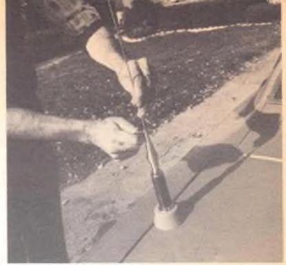
*Insert the whip in the antenna collar and tighten the set screw. NOTE: Most antennas will require tuning with an antenna bridge to operate with maximum efficiency.*
