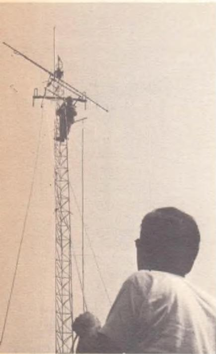
When working on any antenna tower a safety belt is a must.
