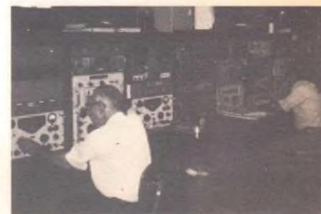
*Operating positions at the Grand Island monitoring station. Note the three receivers, tape recorder, frequency measuring equipment and other instruments available to each operator.*
