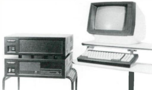
CompuSonics created the DSP-2002 for professional radio and television broadcasting service. Functionally, the DSP-2002 equals or exceeds conventional tape recorders with the additional benefits of digital sound quality, random access and interactive editing. Recording time capacity ranges from 30 to 960 minutes in stereo, depending on the number of Storage Modules installed.
