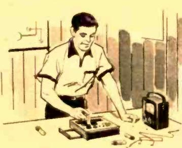
This versatile, low-cost checker tests cathode emission and shorted elements — also continuity.
