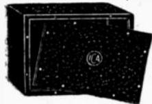
Removable front and back. Spot welded corners. Finished in black wrinkle enamel.
