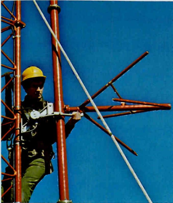
Rigger installing deicer cables on a tower, with insulated guys.
