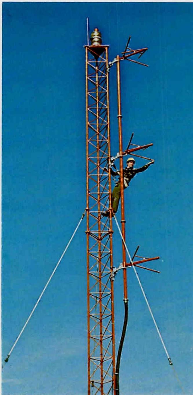
Rigger field tuning a JSCP-3 antenna. Note electrical deicers and insulated guys.
