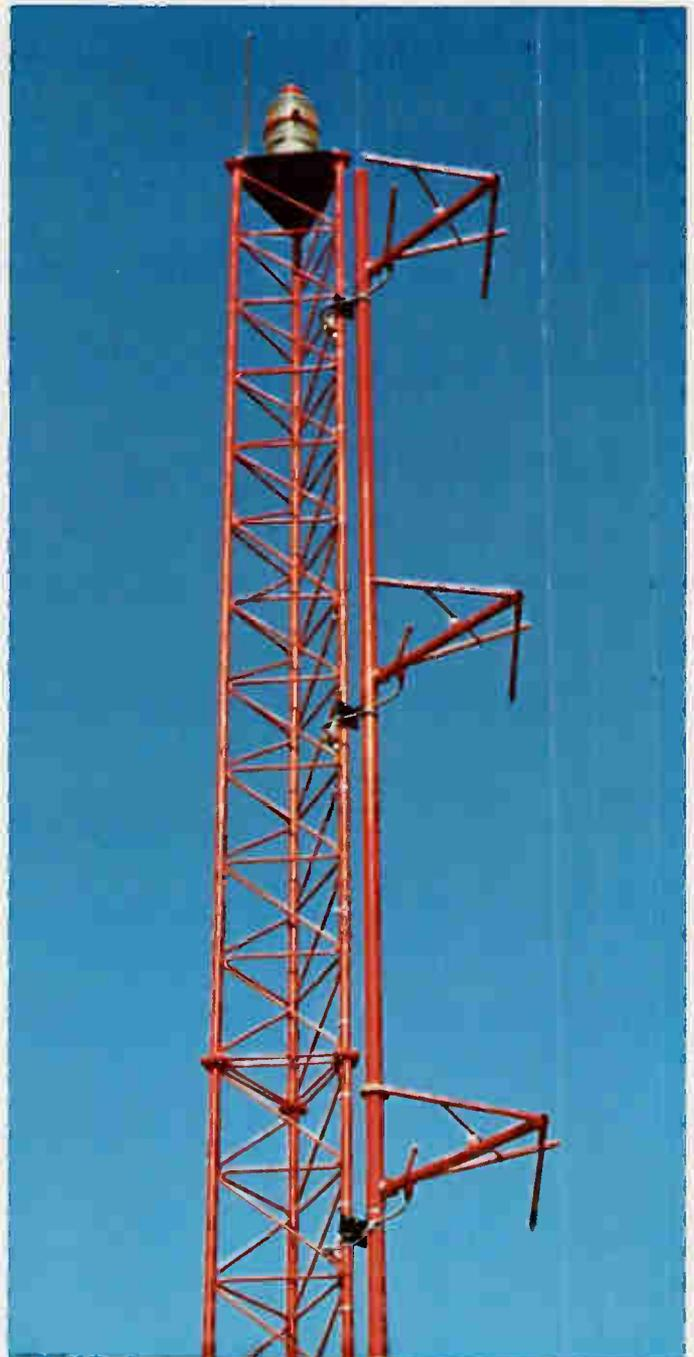
JAMPRO JSCP 3 bay shunt fed antenna using 3/8" rigid line. Note deicer cables.
