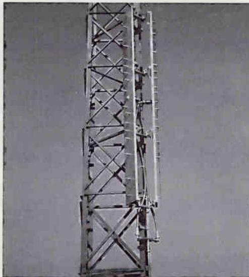
Directional antenna with panels leg mounted to a square tower.
