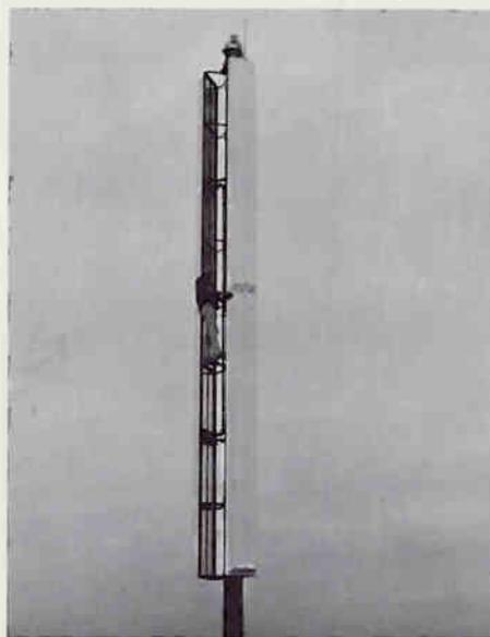
**Deicing radomes placed over four panels of a directional zig zag antenna.**
