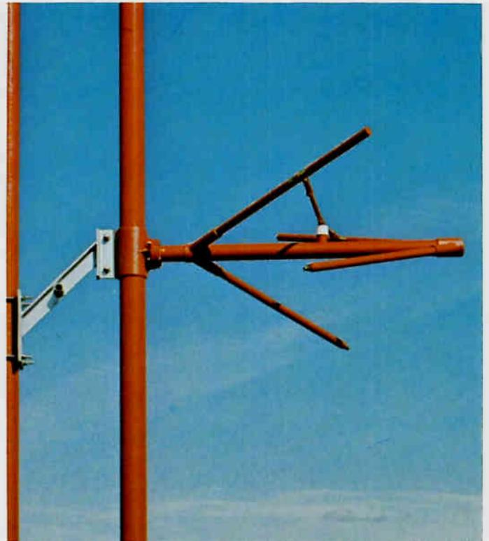
Heavy one piece casting holds coax line and element to bracket for typical leg mounting.
