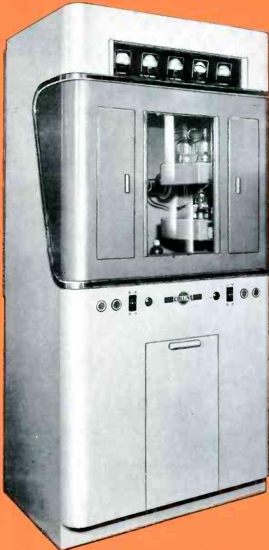
The new 20V is designed for continuous high fidelity broadcast operation at any specified frequency in the band from 540 to 1600 kilocycles or any of the high frequency broadcast bands up to 18 mc.
