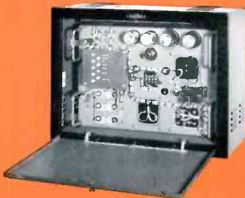
**409U-1 CONSOLE POWER SUPPLY** . . . is a wall mounting power supply for the 212A and 212B series consoles. It contains three supplies which furnish d-c power for preamplifiers, monitor and line amplifiers, and 12 volts for relay operation. In addition, it furnishes 6.3 volts a-c to operate all tubes in the console.
