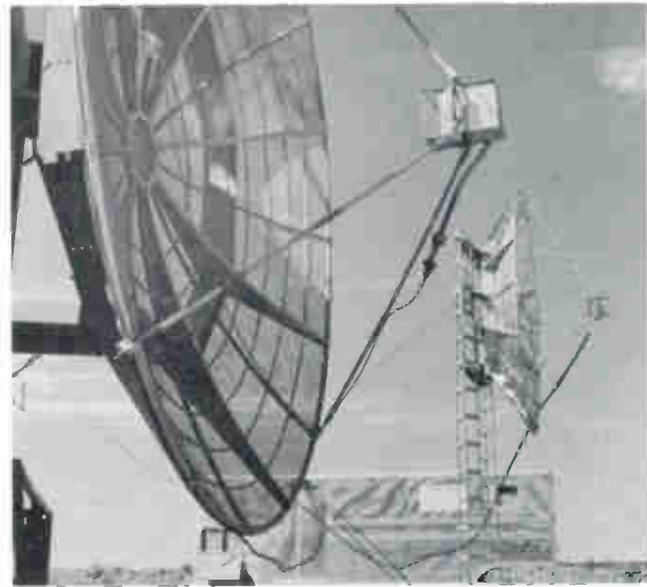
PROPAGATION STUDIES, by such means as this transportable terminal, have aided in application of scatter techniques for reliable communication.
