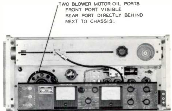
Figure 5-1. R-F Unit Blower Motor Lubrication Points
