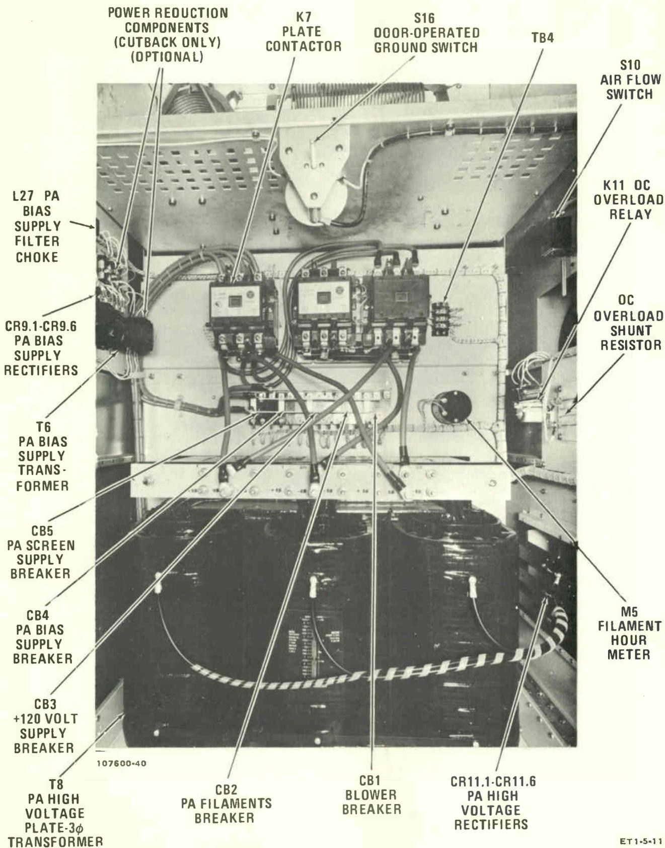
Figure 5-11. High Voltage Plate Transformer and Bias Supply, Lower Left-Hand Compartment, Viewed from Rear
