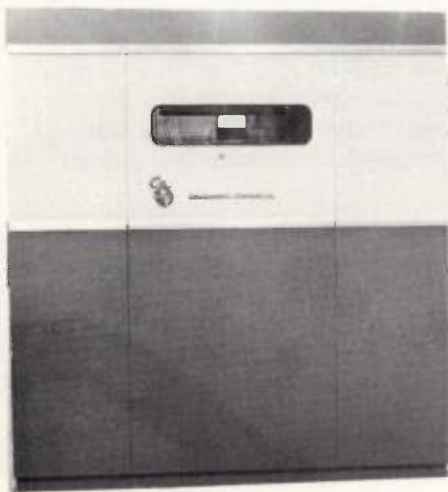
Continental 100 kW combiner is used to combine the output of two Continental Type 317C-2 50,000 watt AM broadcast transmitters.
