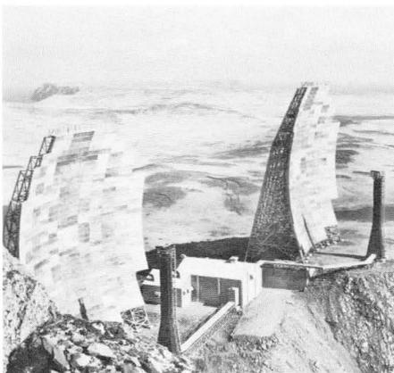
On the Cover—120-foot antennas used at one of the tropospheric scatter sites in the Aleutian Islands. This is one of the many tropospheric scatter installations using Eimac power amplifier klystrons. The transmitters at this site were manufactured by Radio Engineering Laboratories, and the installation was engineered and directed by Western Electric Company.
