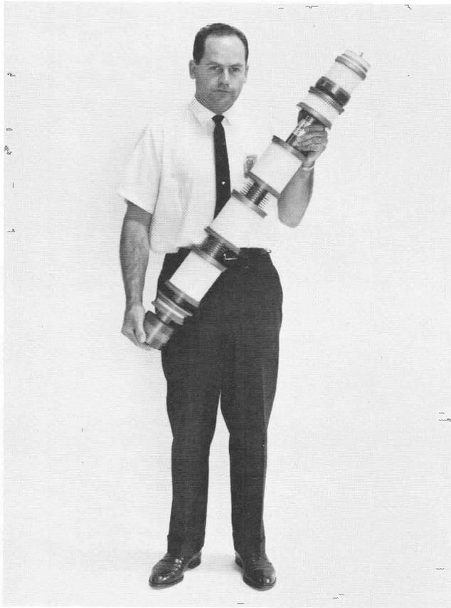
Figure 11—Recommended Method of Hand Carrying Eimac Klystrons.
