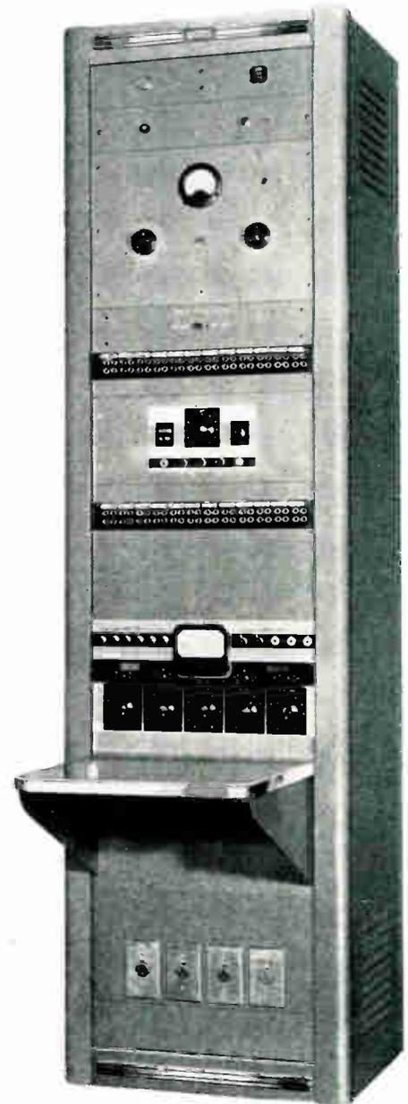
A new station in Pennsylvania got the above cabinet of equipment along with others of a completely co-ordinated factory wired installation. This type is different than the 5M but is shown here as one example of what can be done to supply a tailor-made installation to exactly fit your needs. The cabinet contains complete audio facilities for the transmitter installation to supplement those of the studios.
