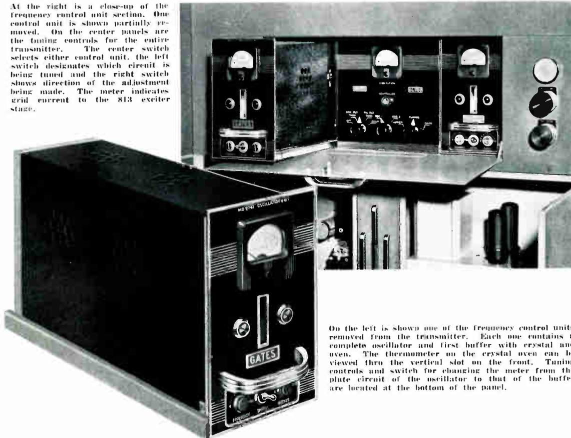
On the left is shown one of the frequency control units removed from the transmitter. Each one contains a complete oscillator and first buffer with crystal and oven. The thermometer on the crystal oven can be viewed thru the vertical slot on the front. Tuning controls and switch for changing the meter from the plate circuit of the oscillator to that of the buffer are located at the bottom of the panel.
