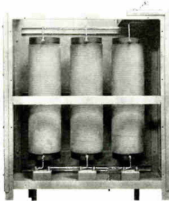
This portion of the 46A equipment contains the tower lighting chokes.
