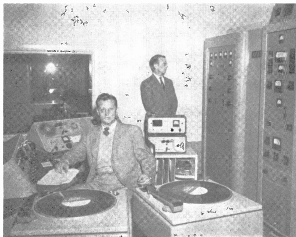
Complete businesslike installation of BC-250GY transmitter and associated equipment is well illustrated in this photograph from KPAT, Pampa, Texas.
