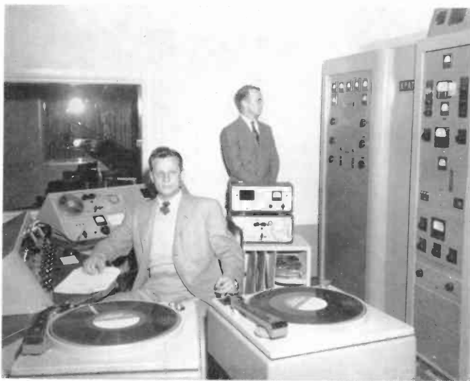
Complete GY-48 Radio Station with Gates Speech Equipment at Radio State KPAT, Pampa, Texas. Note massive appearance and excellent combination type installation.
