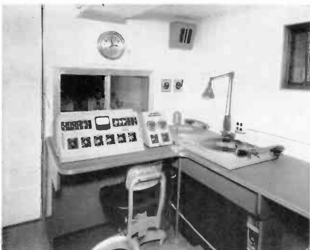
Below, to the left, 52-CS studioette in mobile radio studio supplied to the United States Government. Right, a typical studioette installation with tape recorders and turntables.
