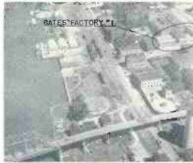
Gates Plant No. 1 On Mississippi
