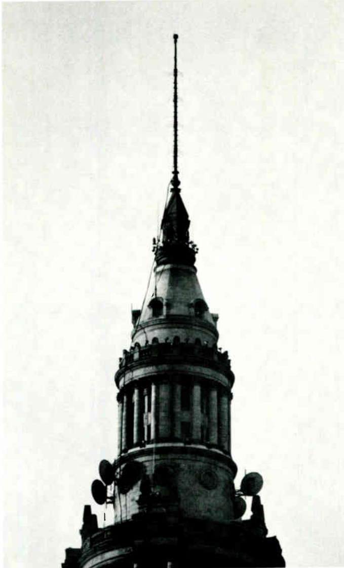
Gates' Directional Dual Cycloid antenna, installed at Station WCLV-FM, Cleveland, Ohio, is mounted atop the 640 foot Terminal Tower Building in downtown Cleveland. The WCLV-FM antenna consists of four Gates' directional circularly polarized elements. This antenna is available in arrays with up to eight bays.
