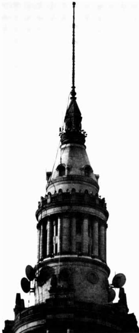
**Gates' Directional Dual Cycloid antenna, installed at Station WCLV-FM, Cleveland, Ohio, is mounted atop the 640 foot Terminal Tower Building in downtown Cleveland. The WCLV-FM antenna consists of four Gates' directional circularly polarized elements. This antenna is available in arrays with up to eight bays.**
