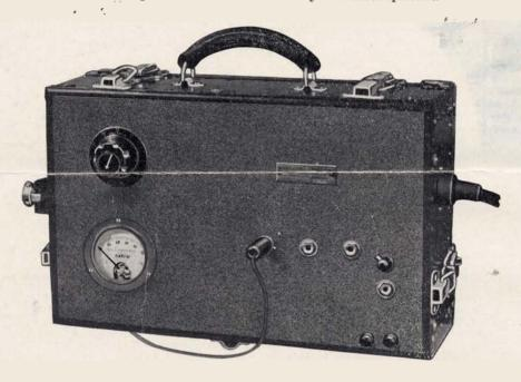
The Model B-60 Remote Amplifier is the last word in true high fidelity moderate priced remote equipment. It is now in use by stations of the 100 watt class and of the 50,000 watt class and is continually bringing unsolicited comment from users as to its real construction and performance.
