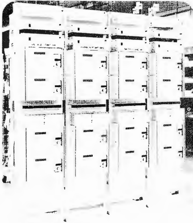
Typical FV8F protected IF repeaters
