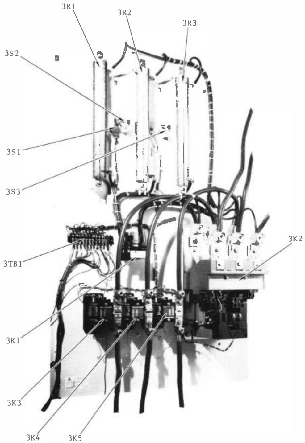
Figure 2-16. High-Voltage Step-Start Assembly
