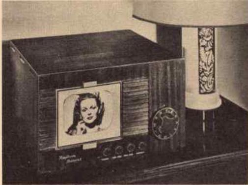
This beautiful 18 tube television receiver built by Belmont Raytheon uses a 7JP4 direct view picture tube. The five panel controls are station selector, volume and off, vertical hold, horizontal hold and contrast. The tuner covers all 12 TV channels. The audio portion uses FM for maximum quality sound.
