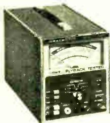
Designed for TV use, this portable meter easily checks yoke windings, flybacks, horizontal coils, and 10 kHz to 100 kHz general purpose coils. Good/bad ring test with  $\pm$  1 ring accuracy at 10 mark on highest range. Also measures TV voltages up to 300 V peak-to-peak (up to 40 kV
