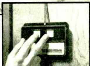
Two-button safety wall switch prevents accidental door movement
