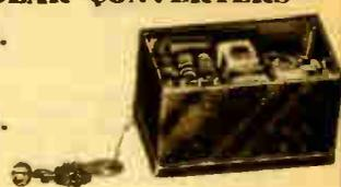
A.C. Radio Receivers may be operated from 32 or 110 volt D.C. source by means of this new device. Magnetic type with no moving parts to create interference. Compares very favorably with motor generators and their efficiency is considerably greater. Does not increase hum level of receiver. Magnetic unit will give over 1000 hours of service and can be replaced as easily as a radio tube. Size, 1 1/2 x 6 1/2 x 6 1/2 Ins. Shpg. Wt., 16 Lbs.
