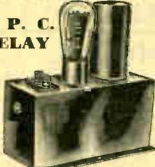
Suitable for any of the uses to which an extremely sensitive photocell relay may be put. Capacity 25 watts, non-inductive load. Adjustable for any desired light value. Operates normally open or closed. Requires standard photocell and -12A radio tube for operation. For either 110 volt A.C. or D.C. as specified in ordering.
