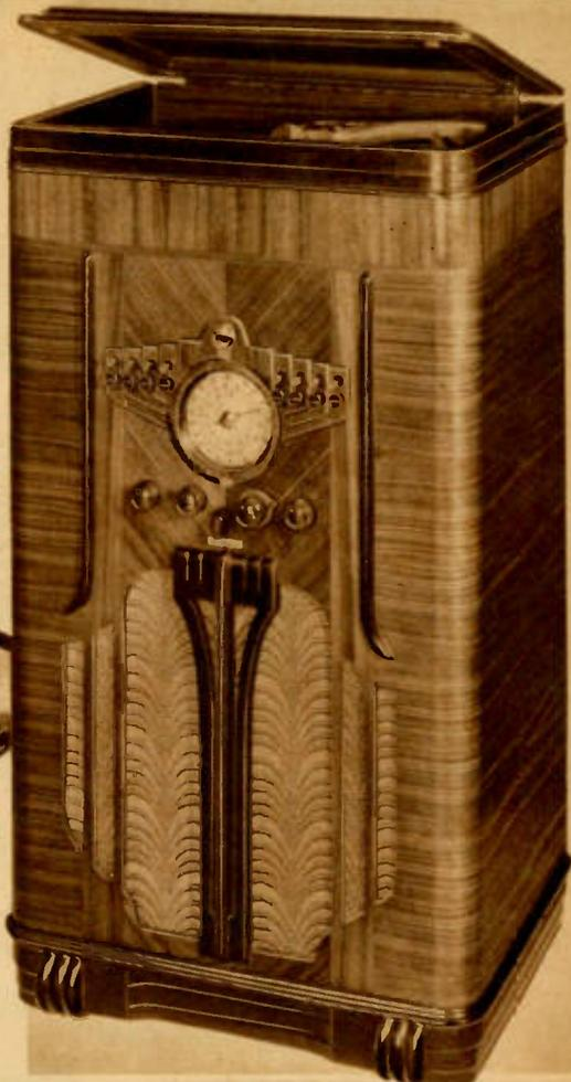
The superheterodyne features, in addition to the sensational Touch-Tuning (fully described on page 20) such other advancements as a tone expander which, by means of a high fidelity switch, permits reception of all of the sidebands, lost on ordinary receivers.
