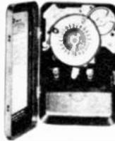
Turns equipment "on" and "off" once in 24 hours, or from 1-12 "on" and "off" operations a day can be obtained by use of extra trippers—can be added without removing dial. Min. on or off time 1 hr., max. 23 hours. Can be turned on or off manually with reset SPST switch rated at 40 amps. 4375 watt capacity. Mounting holes and knockouts. Gray steel case. UL approved. Operates on 110 volt 60 cycle AC. 7¾Lx5Wx3"D. Shpg. wt., 4 lbs.
