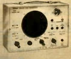
MODEL 802 SIGNAL TRACER AND GENERATOR KIT. Combination signal tracer and generator. In the absence of a signal it generates its own signal for audio, IF or RF testing. Incorporates a noise locator circuit for checking noisy components. Provisions are made for using the instrument as a substitute speaker or amplifier. Audio Freq., 400 cycles; IF Freq., 455Kc (Mod.). Complete with demodulator and audio probes. 10"x7"x5". Shpg. wt., 8 lbs.
