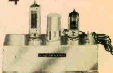
Have fun making announcements and broadcasting music through your own radio—with this broadcaster. Simply connect high impedance microphone or phono pickup to broadcaster and tune in broadcaster on radio. No wiring between the broadcaster and radio set. Pretuned to 1600 on radio dial but easily retuned. With 12BE6 and 35W4 tubes, phono jack, 2 feet of antenna, schematic and line cord. Completely wired. Chassis size: 4x2". For 110-125V AC/DC operation.
