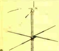
Isolating skirt for use with Citizen's Band Ground Plane Antenna HE-66WX. Mounts 9 feet (1/4 wave length) below ground plane (i.e. 27 MC). Lowers angle of radiation and minimizes effect of mounting structure. Improves performance of ground plane. Clamps to 1 1/4 inch tubing or 1 inch pipe. Shpg. wt., 4 lbs. HE-681WX ..... Net 11.14
