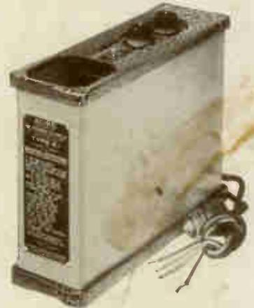
The Acme B Eliminators have no hum and what's more no distortion. When high B battery voltages (up to 180 volts) are used and where constant and uninterrupted service is required use this eliminator. The Raytheon tube is included and has no filament to burn out. A F, R F and detector voltages are available.
