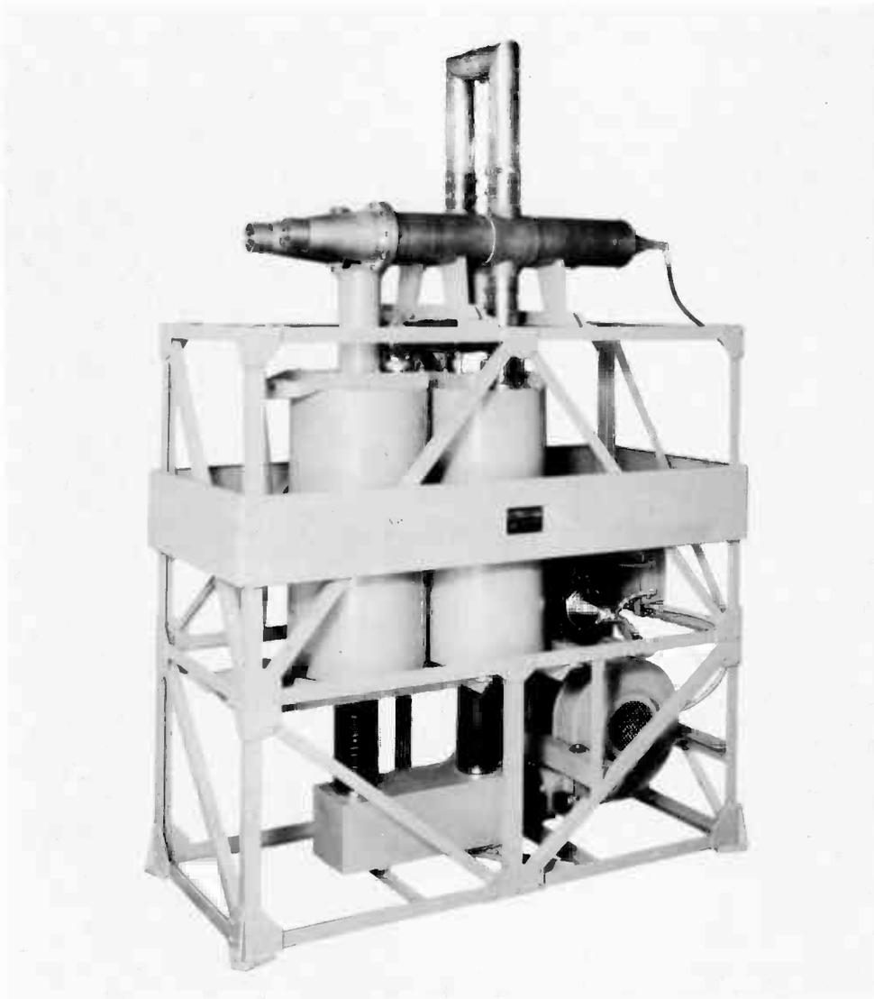
**Type 1052 Diplexing Filter, Channel 12**
