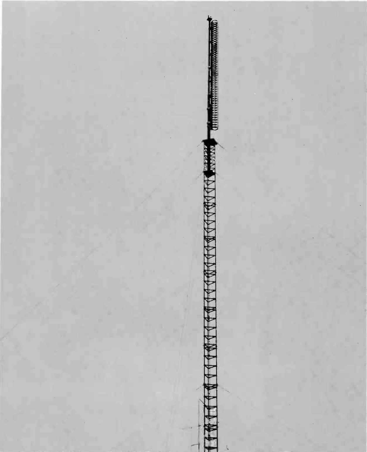
A one-bay Type 1046-N Antenna Array after installation at Station CHEK-TV, Channel 6, Victoria, British Columbia.
