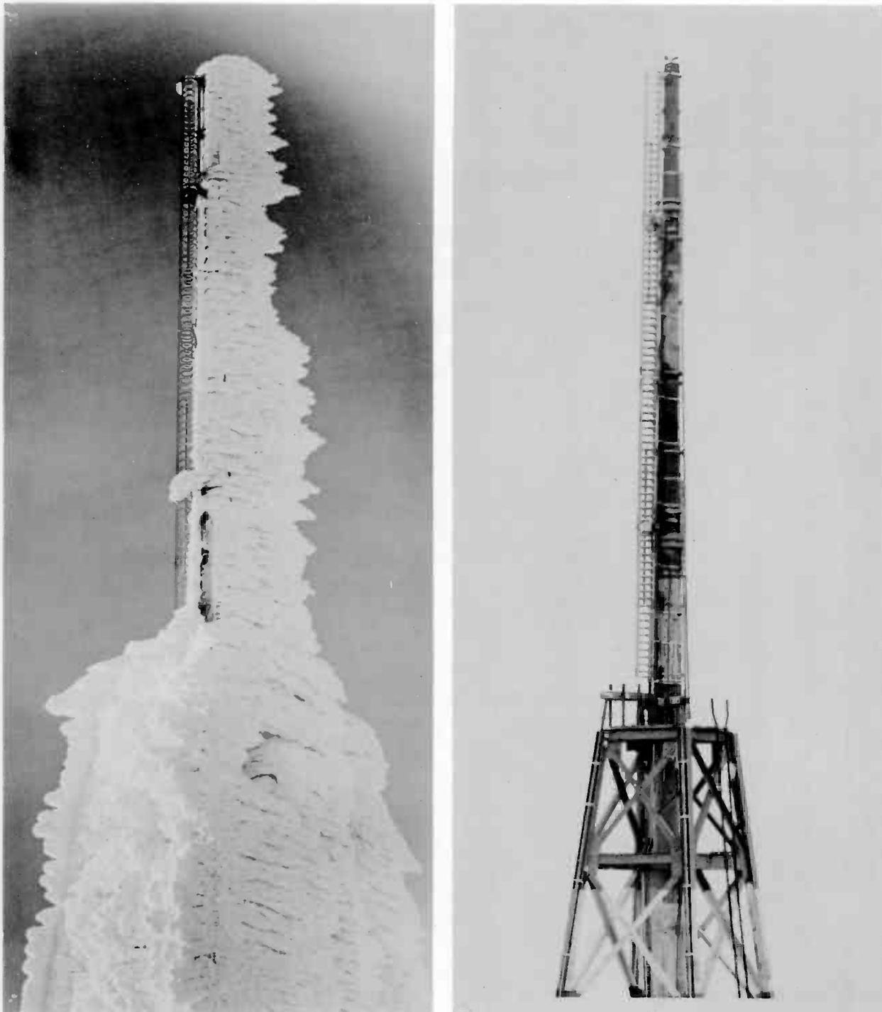
Two views of the AMCI Two-Bay Type 9900 (a special type with extra deicing capacity) Antenna Array at Station WMTW (TV) Channel 8, on Mount Washington, New Hampshire. Picture at left was taken after a typical sleet storm and shows the antenna itself completely deiced. (The mast and tower are not intended to be deiced.) The quality of the televised picture remained normal.
