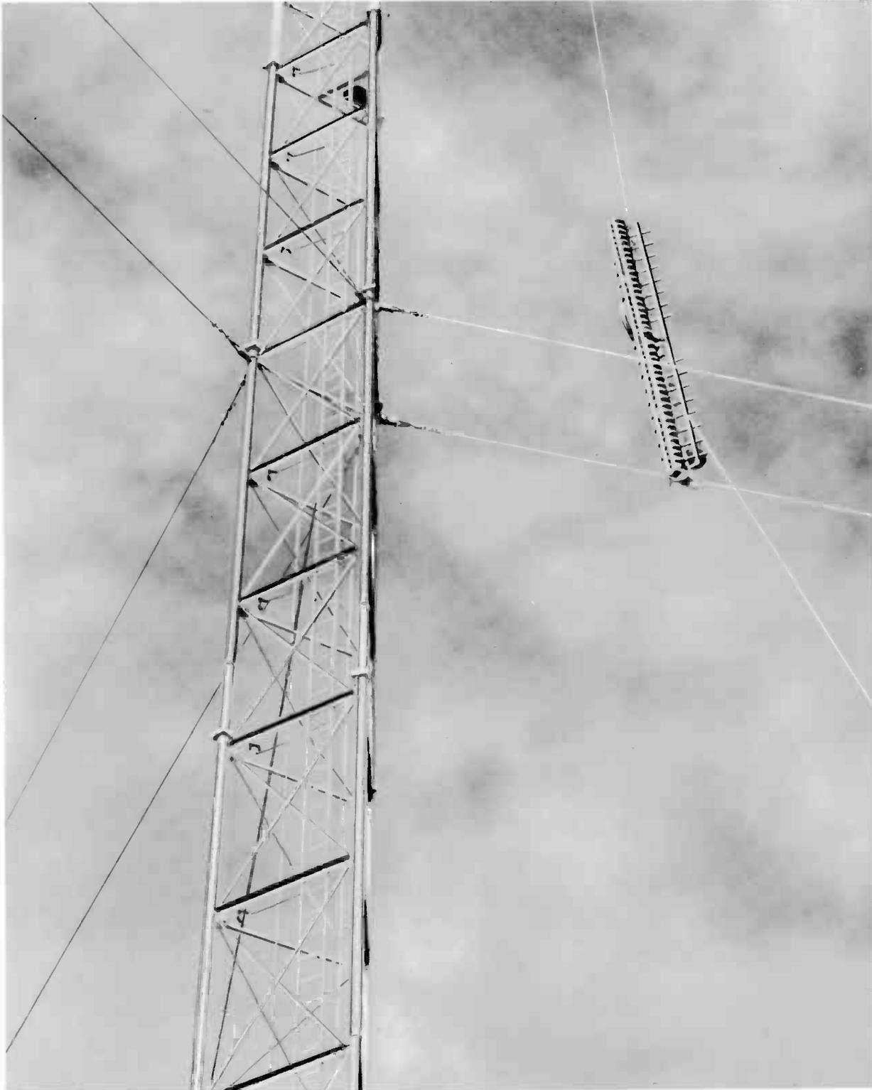
Shown above is a portion of a Three-Bay Type 1030S Directional Antenna Array with Type II Null Fill-in during its installation at Station CJLH-TV, Channel 7, in Lethbridge, Alberta, Canada. The maximum gain of the array is 20.8. The picture shows one of the directional bays being raised to the top of the tower.
