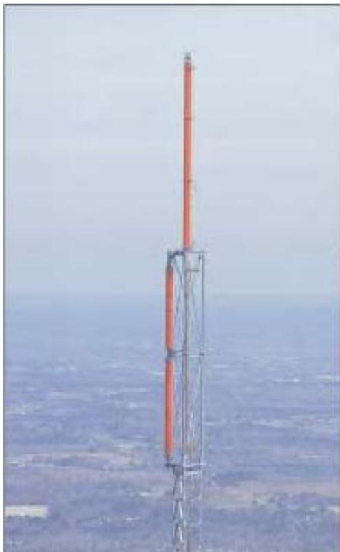
Now Andrew offers a unique solution (patent pending) to the problem of diminishing tower top real estate. The STACKER offers high antenna density without the tradeoffs of in-line stack designs or the expense of a Candelabra or T-Bar.
