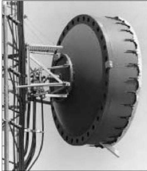
Multiband antennas offer very high route capacity at minimum antenna/tower system cost. They also offer great system planning flexibility, especially for upgrades of existing frequency congested routes. Multiband antennas provide a second frequency band of operation using one antenna. Maximum channel expansion, with minimum increase in tower wind load, saves system installation time and cost.
