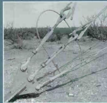
Andrew guyed towers use flexible anchor shafts to dampen guy vibrations caused by wind gusts.
