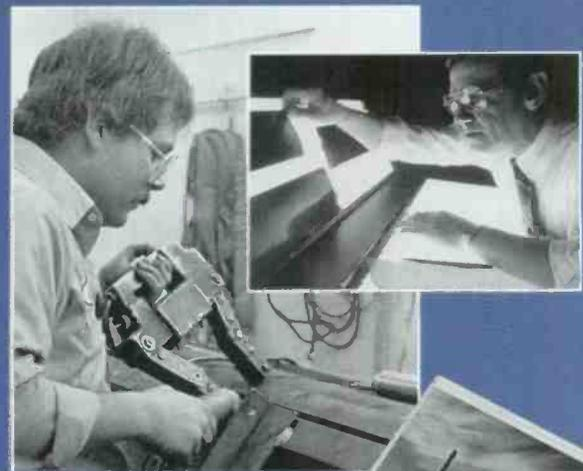
All welding is performed by certified personnel and checked by Quality Assurance. Above Magna flux testing; above right X-ray results being checked.
