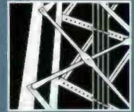
Support channels are mounted at 4 foot (1.2 m) intervals inside, outside or on both sides of one or more tower faces. The supports are provided with 7/16 inch holes for mounting standard HELIAX® cable and elliptical waveguide hangers and with 3/4 inch holes to accommodate Andrew snap-in hangers.
