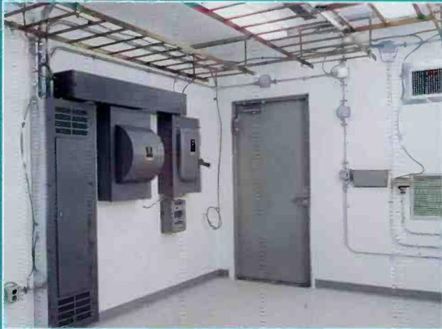
In addition to the basic electrical components, this electrical system features an array of options including a manual transfer switch, a surge arrester, a safety switch, alarm cabinets, emergency lighting, a power failure alarm, a door alarm, and timer. Halo ground systems are installed with ground drops, pigtailed for on-site connection.
