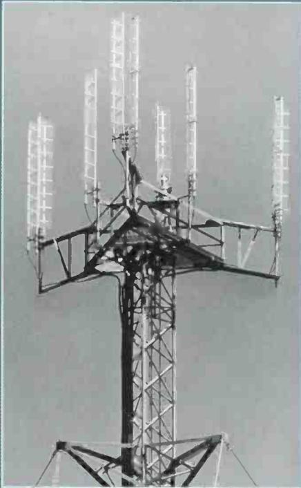
Cellular platforms provide a safe and easy access for antenna installation. Maximum antenna separation is achieved by adding retractable arms.
