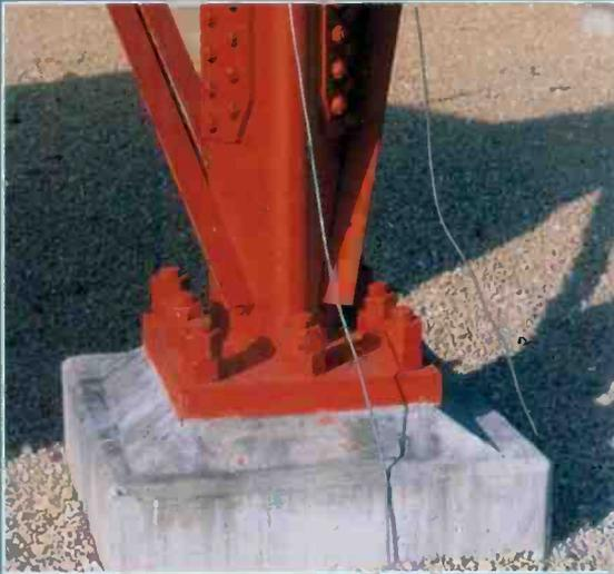
Plate leg members and high strength bolts ensure structural rigidity.
