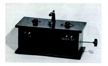
Figure 6 — Station 3BV's receiver. The first model (1910) employed an electrolytic detector. This model, a revised version, employs a crystal detector.
