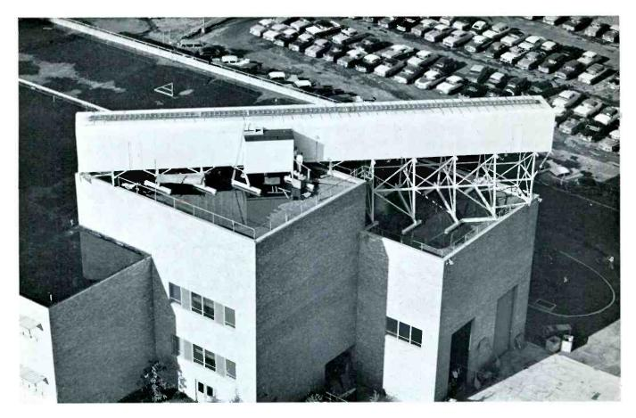
Figure 1 — UHF Linear Array, a complete operating radar, including transmitter, receiver, modulator beam steering circuits and associated controls.
