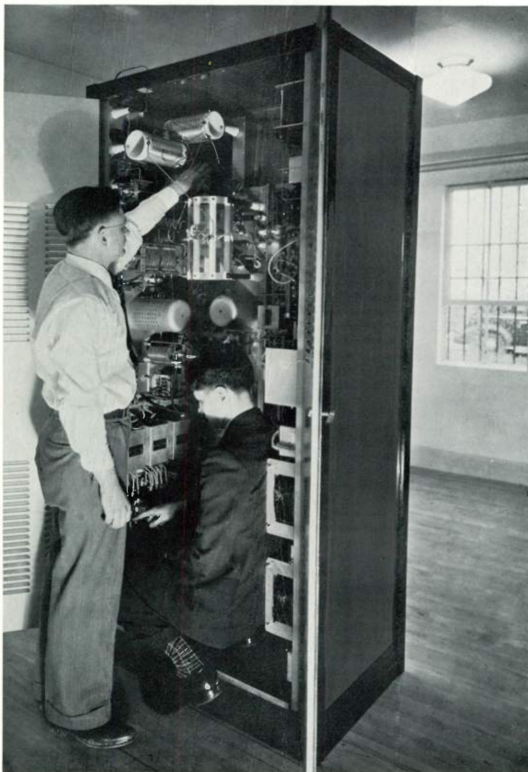
Accessibility of vertical chassis construction is demonstrated during the installation of a 250-D Transmitter at WMBO, Auburn, N. Y.
