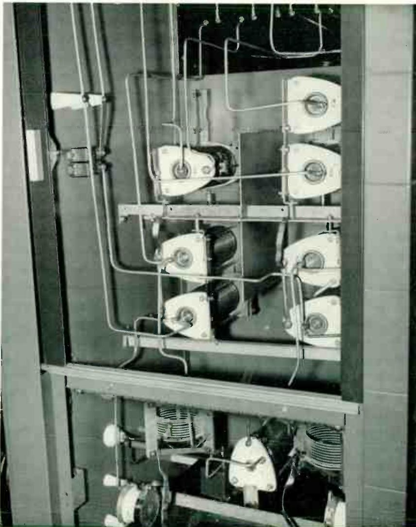
◀ Cabinet at left contains the phasing networks for each of five towers. Each transmission line has its own meter. Note the "twin-ganged" rotary coils used for the series of arms of the phasing network.
