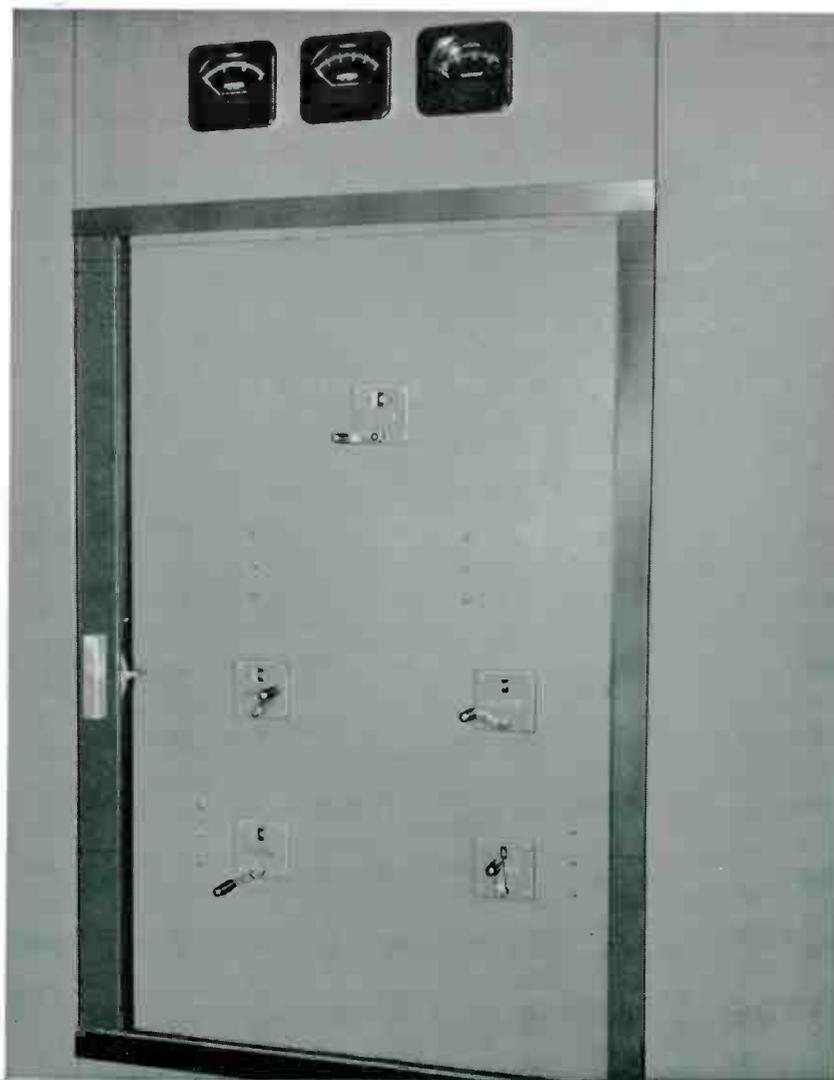
Phasing equipment installed at Radio Station KSOO is housed in the new type horizontal sliding door cabinets. Cabinet at right contains the power and current dividing networks for each tower and day-night pattern-change relay.
