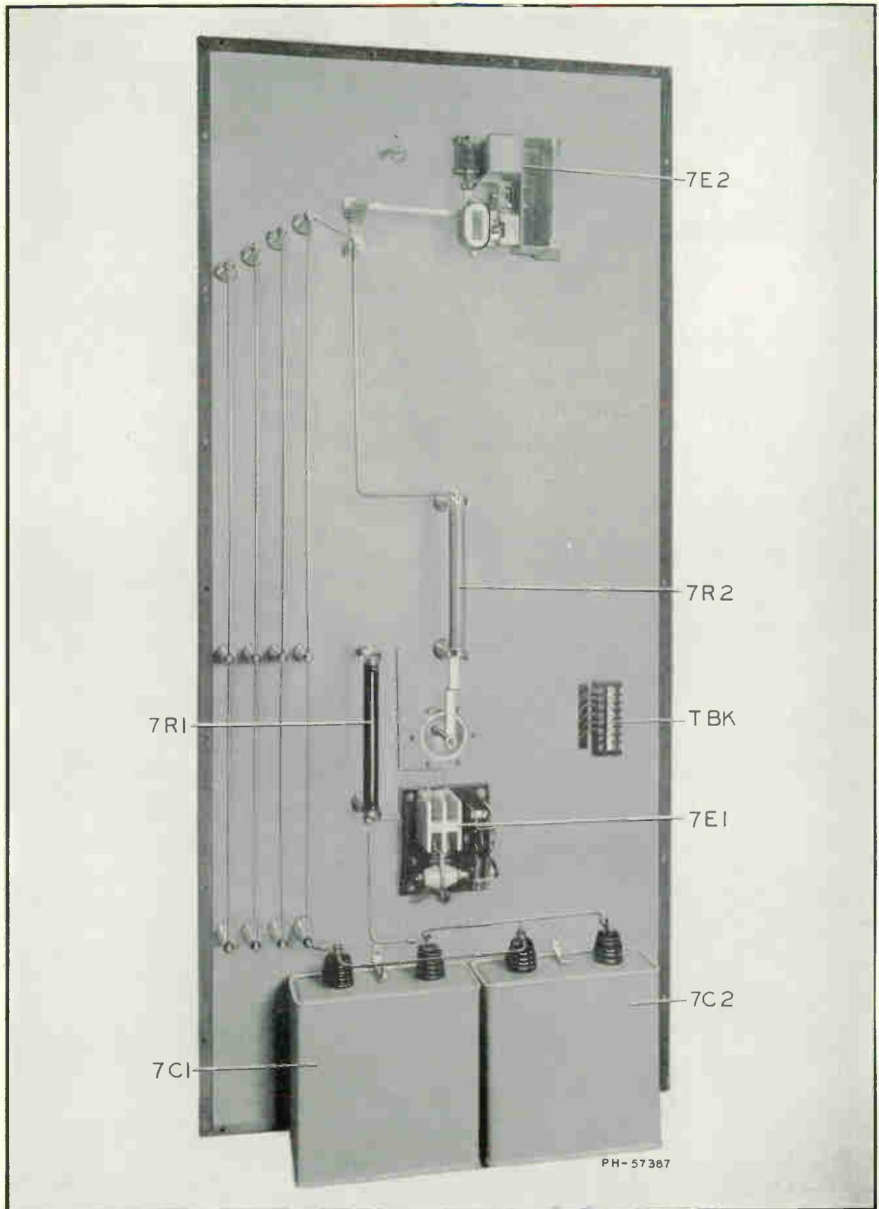
Figure 17—Rectifier Auxiliary Chassis
