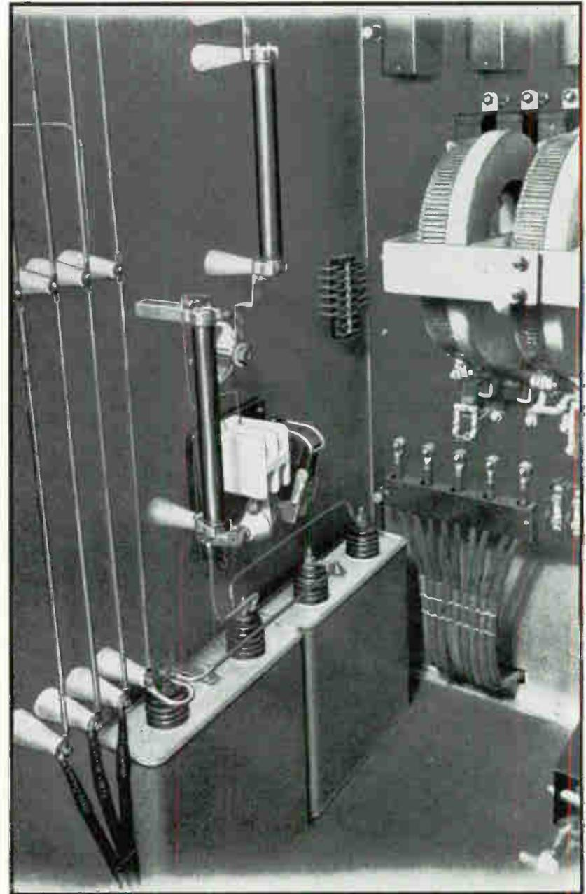
Figure 3—Power Supply Cable Lacing
