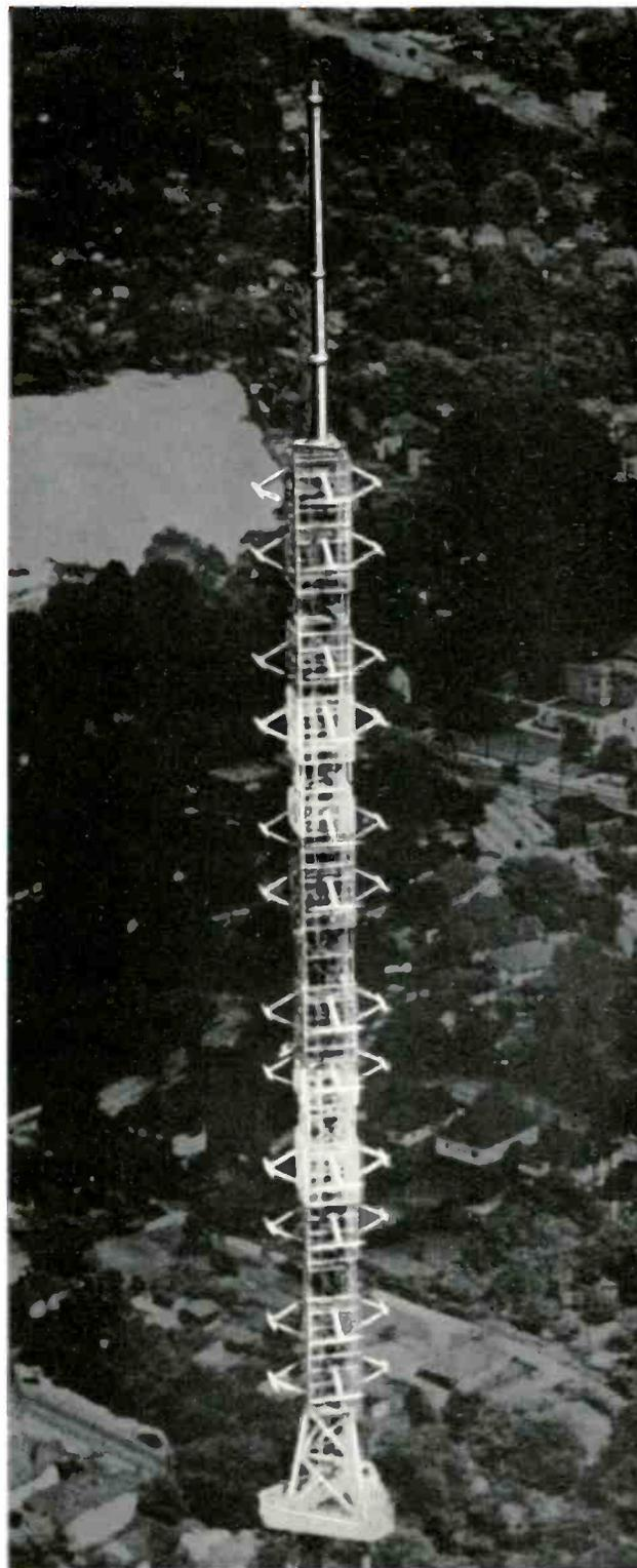
Supergain Antenna at WSB, Atlanta, Ga. Since this photo was made, the antenna has been changed from a 12-section to a 14-section type.
