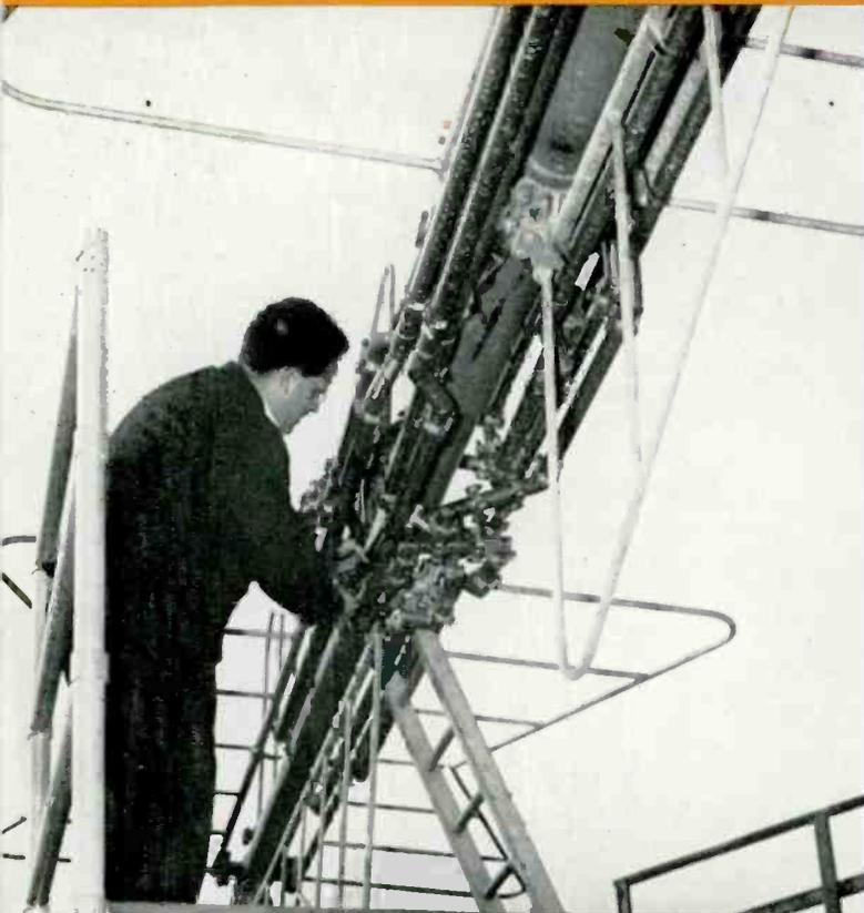
Closeup photo showing the construction of a special copper feedline dress for a custom designed RCA Superturnstile Antenna.
