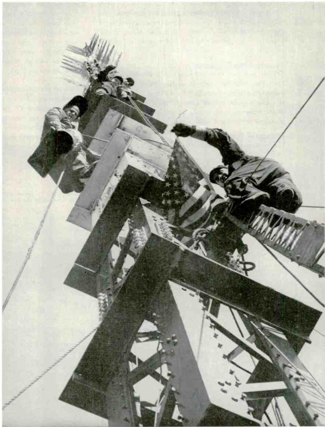
▲ Photo showing a closeup of the "multiple-use" TV antenna supporting tower located atop the Foshay Building, Minneapolis, Minn. The seven diaphragms on lower portion are for strengthening and permit supergain elements to be mounted in between them.
