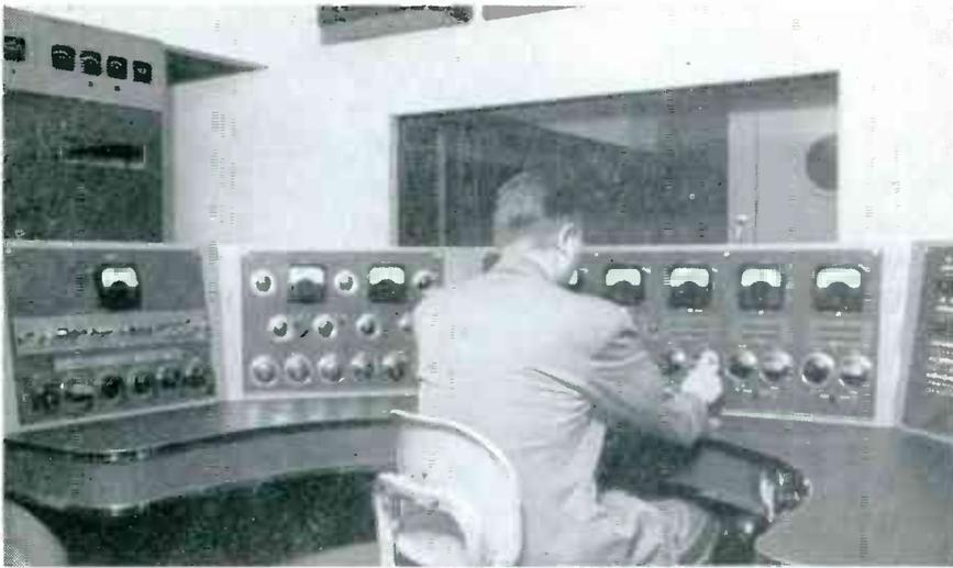
*KOMO, Seattle. This master control console—with 9 deluxe audio equipment racks (at rear, not visible)—is one unit of KOMO's completely new and modern 7-studio system. It incorporates complete center panel switching for 10 studios and 6 outgoing channels (KOMO-AM, KOMO-FM, network plus 3 emergency).*
