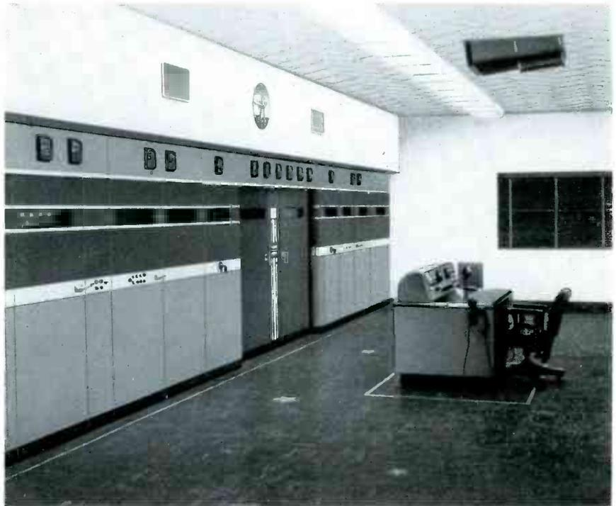
and may be located in the transformer vault or at the rear of the transmitter. A typical transmitter installation requires a space of only 33 x 17 feet for transmitter and associated control and power equipment. A control console finished in umber gray to blend with the transmitter styling is furnished.
