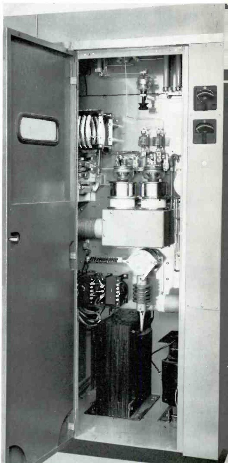
easier maintenance and service. It also permits installation of the transmitter against a side wall, or allows other equipment to be placed on either side of the cabinet. The front doors of the transmitter give immediate access to the front of the vertical panels on which circuit components such as tubes and overload relays are mounted. Remaining components are mounted on the rear of these chassis, while the larger power components are situated in the base of the cabinet.
