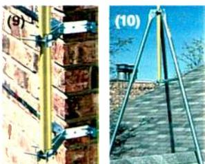
(9) **Corner mounts.** Just the thing for chimney mounting. Two Y-mounts with 5/8" x 10-foot, rust-resistant galvanized straps. 15-527 ..... 11.99
