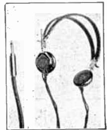
The most sensitive, yet ruggedly constructed unit available. Practically nonbreakable. A 5 foot special moisture-proof cord, with No. 500 telephone type plug attached, and brown leather-covered wire headband with exclusive spring lock and adjusting clamp are all part of this lightweight headset. Dia. 2 1/8", depth 3/4", forged magnet of the best grade 36% cobalt steel. Color... a rich, warm walnut brown.
