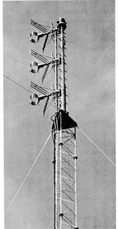
(Right) A Directional FM Antenna, pole mounted, is used by Station WKZN-FM, Kenosha, Wisconsin. Each bay of the directional antenna is equipped with heaters (totaling 900 watts).
