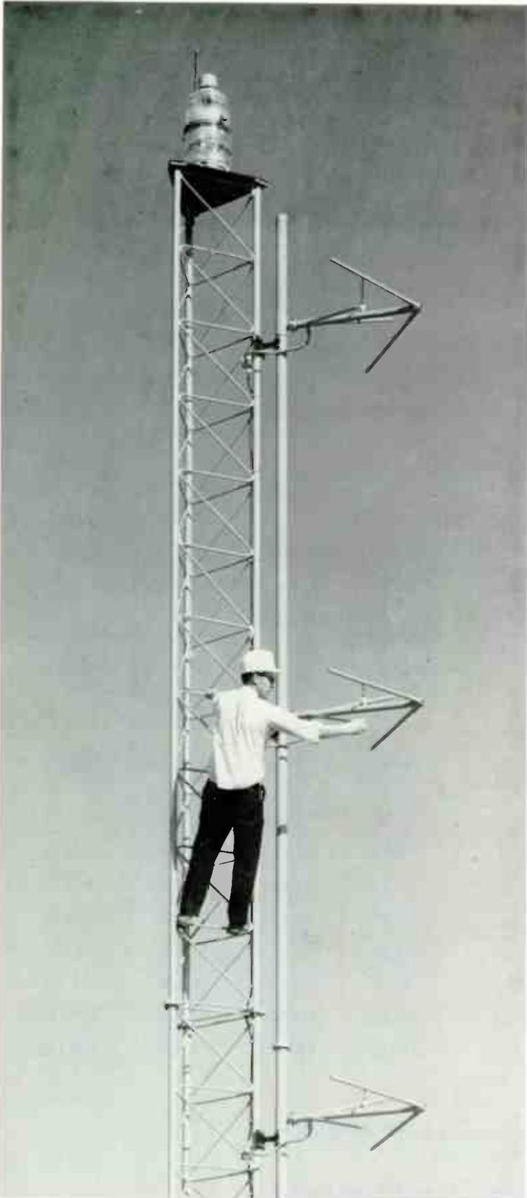
The best state of the art FM transmitting antenna, the JAMPRO CP produces circular polarization by a patented Jampro method.
