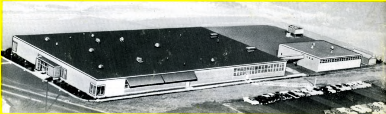
SEMICONDUCTOR MANUFACTURING FACILITY, SLATERSVILLE, RHODE ISLAND
