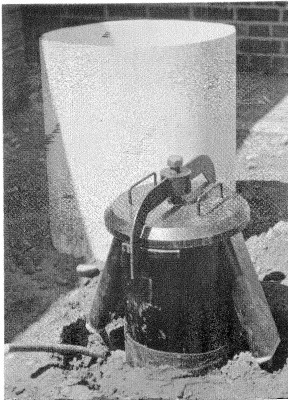
Figure 12—Repeater housing projecting from the ground.
