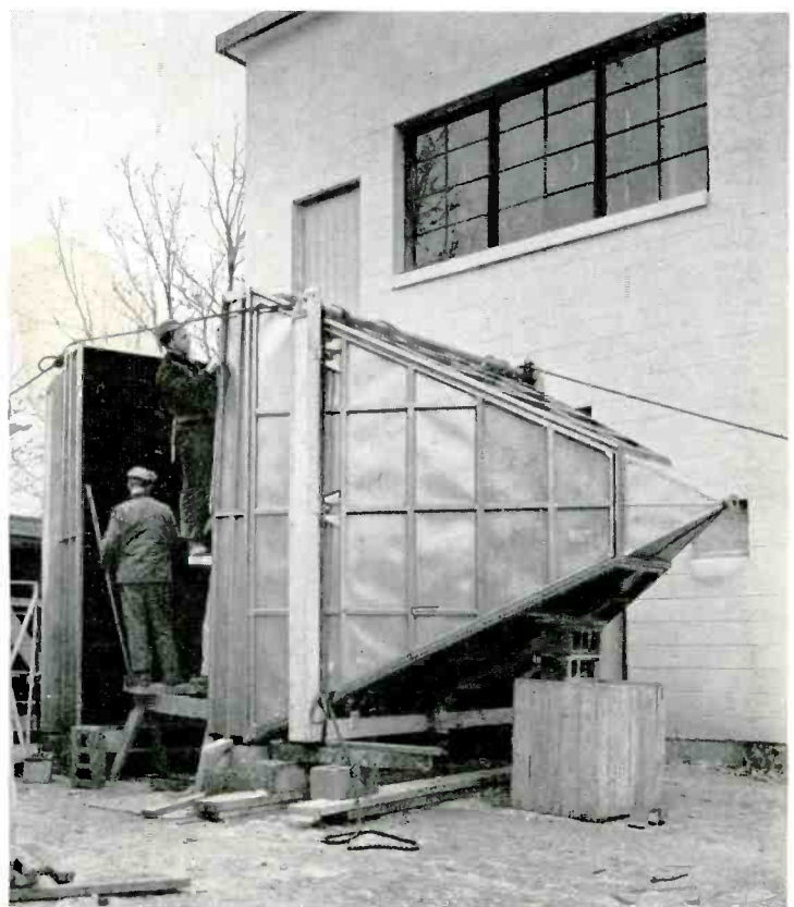
4. Antennas being assembled. By December, these metal lens antennas designed by Bell Telephone Laboratories were ready for hoisting to top of tower.
