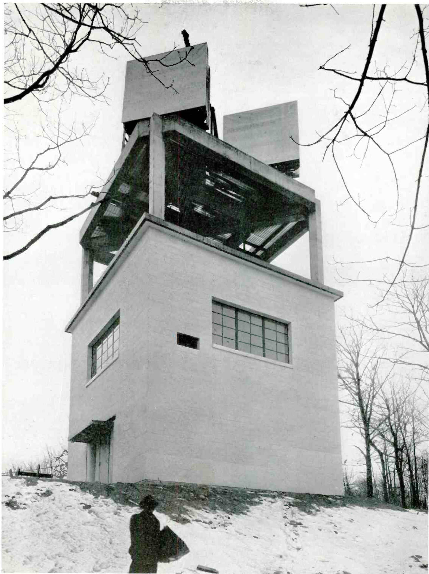
5. Antennas in position. Two of the four metal lens antennas are now in place atop the tower. The next step is the installation of the receiving and trans-
