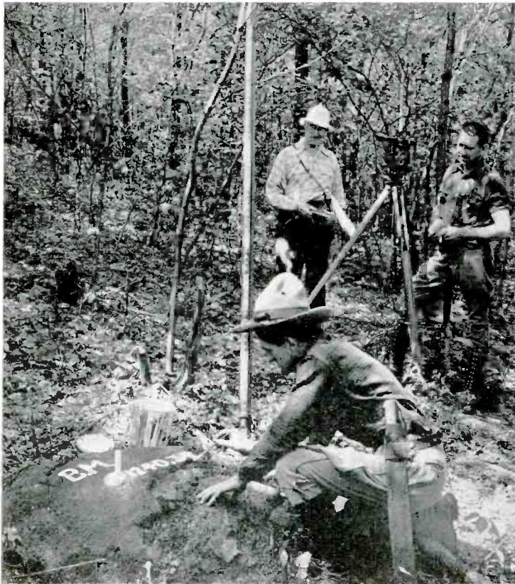
1. Preparation of site. Surveyors establish benchmark on rock at site of first relay station on Jackie Jones Mountain, 6 miles northwest of Haverstraw, N.Y.
