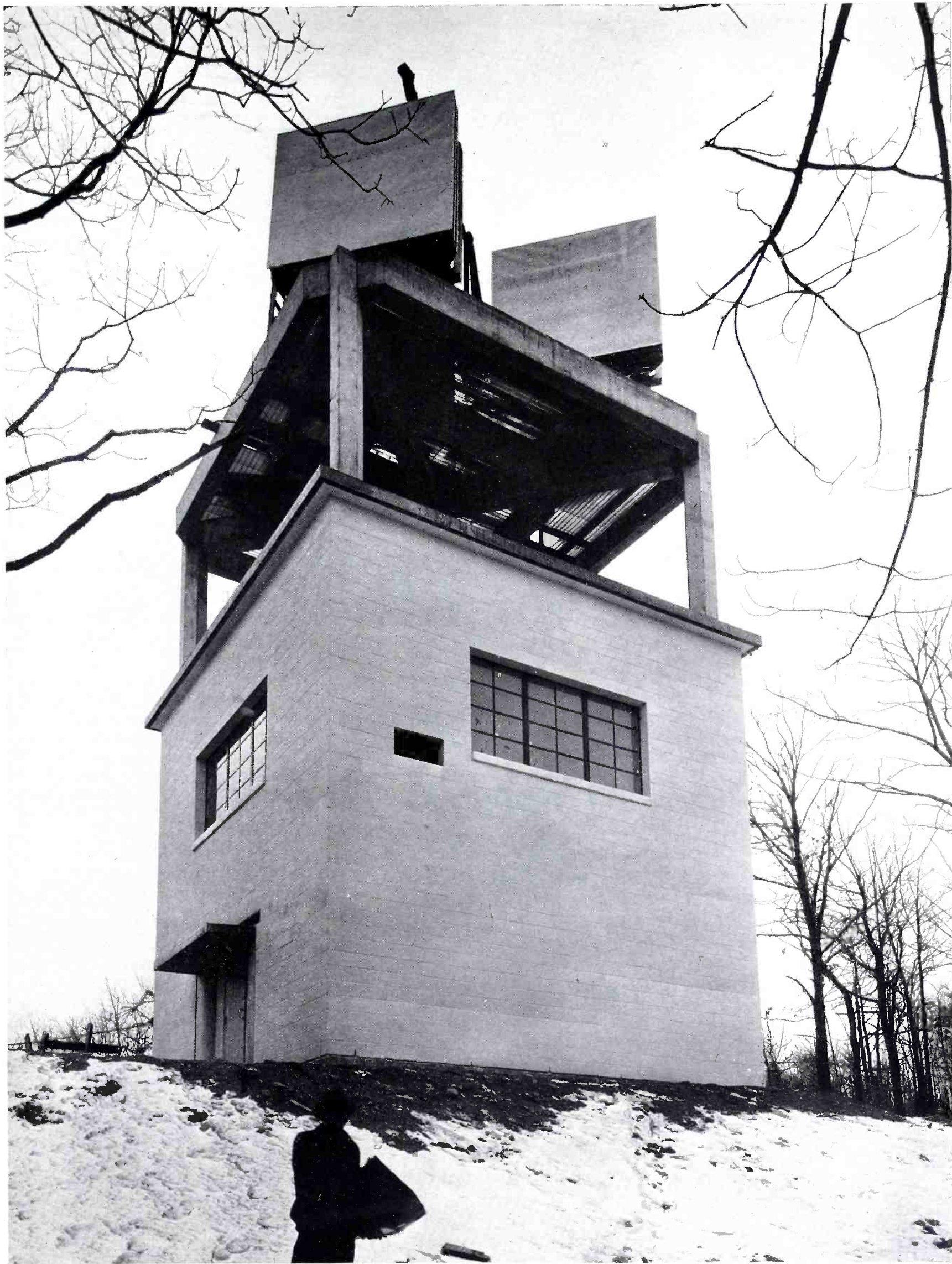
5. Antennas in position. Two of the four metal lens antennas are now in place atop the tower. The next step is the installation of the receiving and transmitting equipment to be completed shortly. Translucent sheets of plastic can be seen covering the lenses of the antennas to provide protection from the weather.
