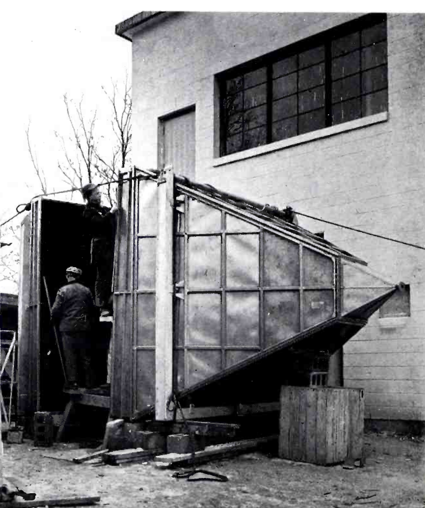
4. Antennas being assembled. By December, these metal lens antennas designed by Bell Telephone Laboratories were ready for hoisting to top of tower.
