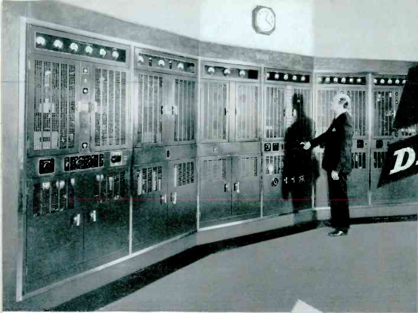
Gordon R. Windham, Chief Engineer, at the panels of 5 KW Transmitter. The two panels at the right comprise a Western Electric 1 KW Transmitter used for standby
